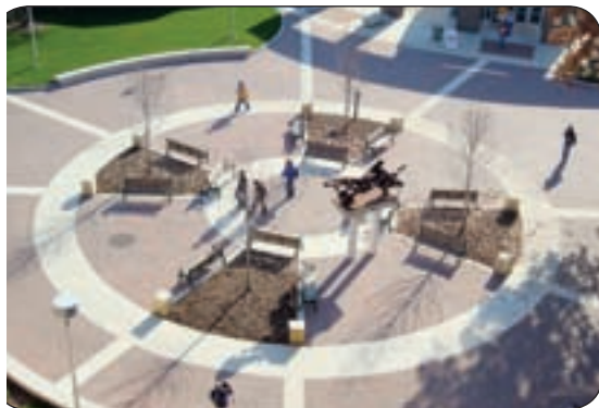
UNI, a watershed landowner, has implemented storm water management practices, including permeable pavers.
