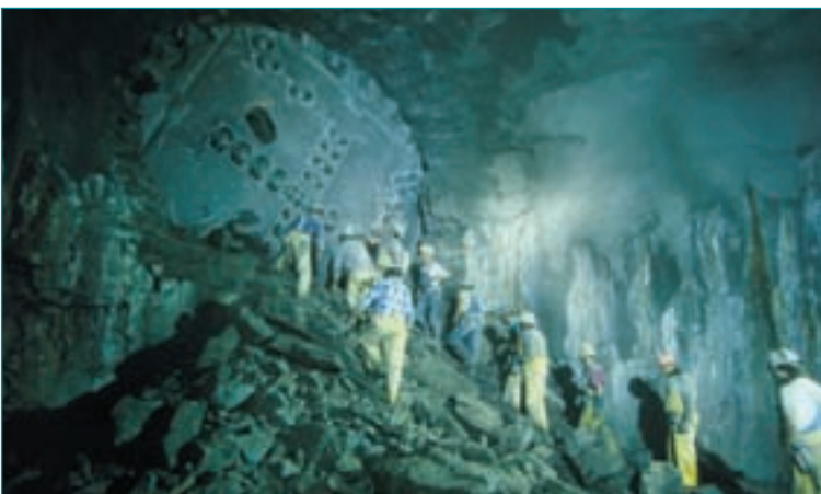
Workers will implement MWRDGC's TARP in two phases.
