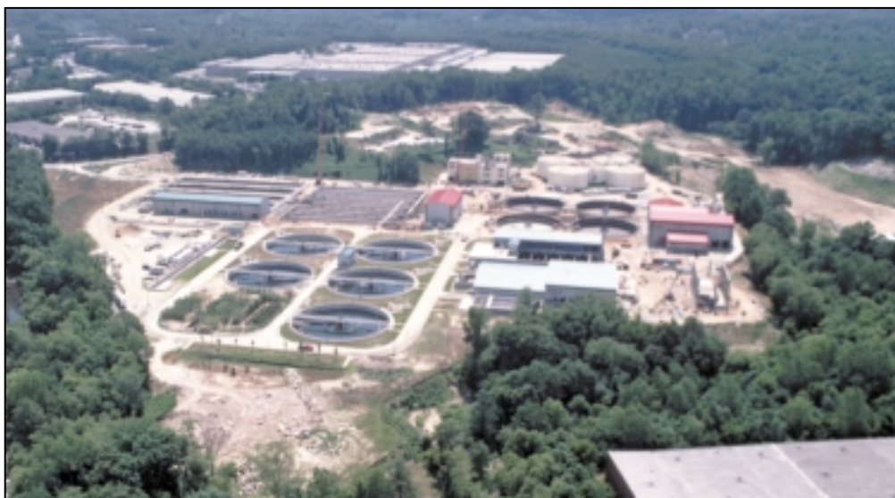
Utoy Creek Water Pollution Control Facility (WPCF). ▶
