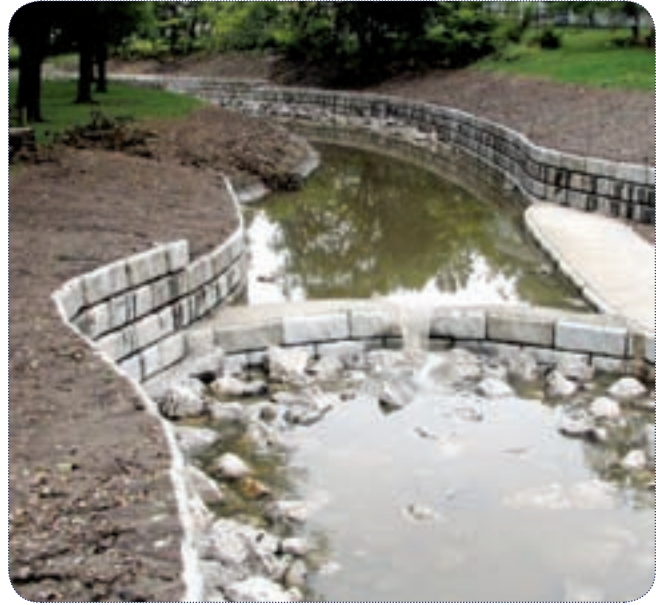
Construction workers installed approximately 38,000 sq ft of retaining walls on site.
