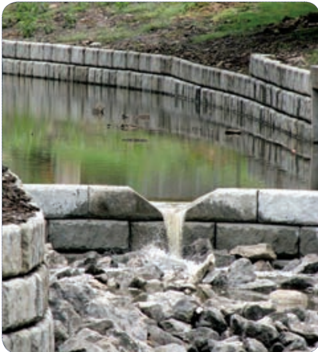
Engineers designed the walls to withstand sporadic water flows and keep off private property.
