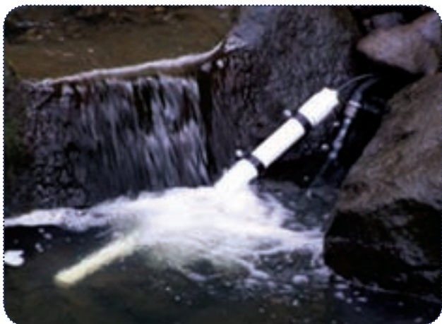
Stations monitor pH, temperature, dissolved oxygen, specific conductance, turbidity and water level.
