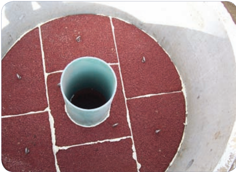
Autosamplers will monitor treatment progress and effectiveness.
