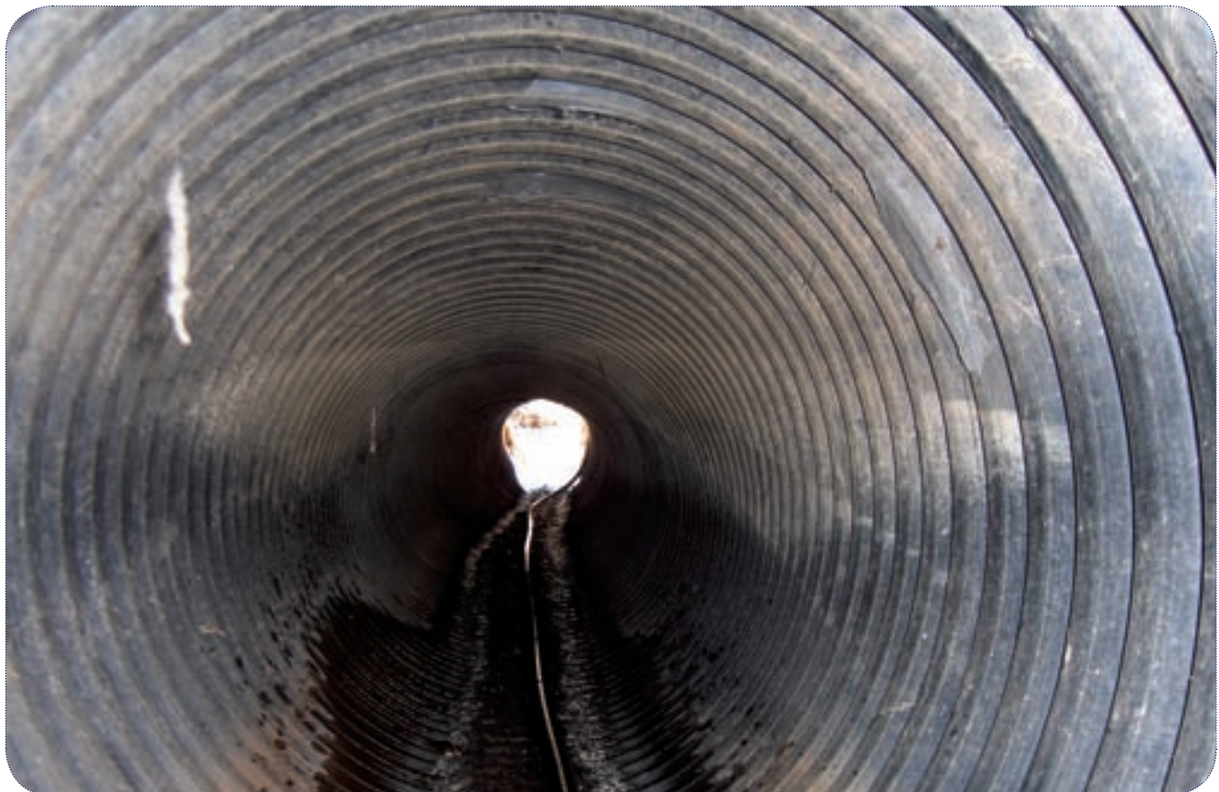
Recent inspections have found no changes in pipe deflection.
