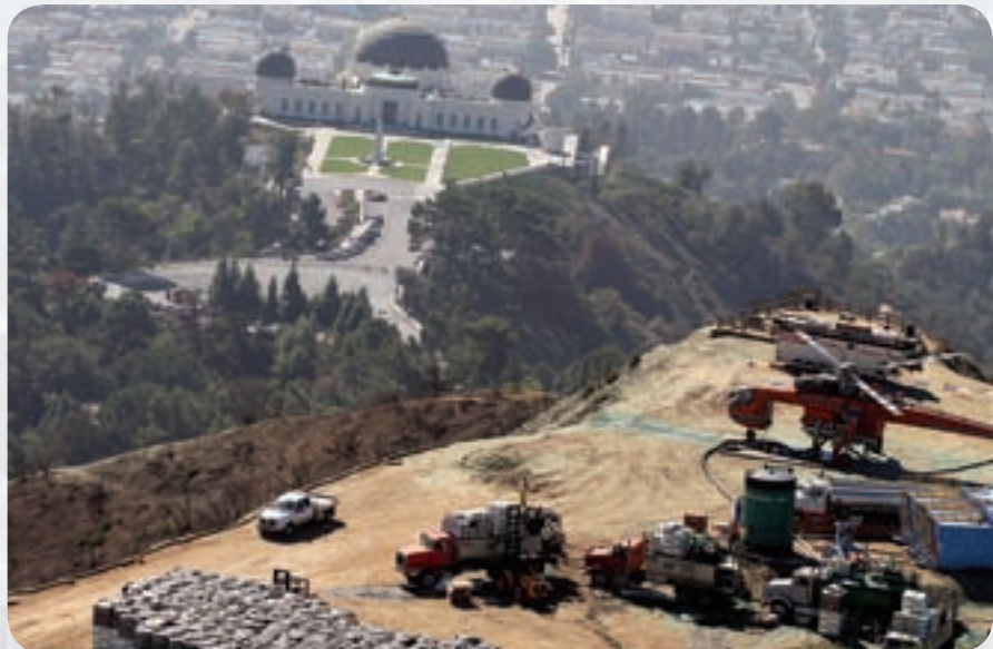
Team members performed assigned loading, mixing and operating tasks in sync to achieve a successful hydroseeding application.
