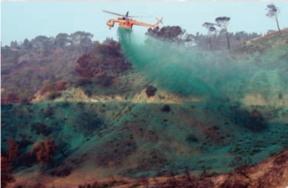
Steep slopes and inaccessible terrain were among the reasons project leaders opted to apply soil stabilization products aerially.
