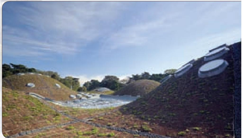
*An intricate system of gabion curbs intercepts runoff, preventing erosion.*
