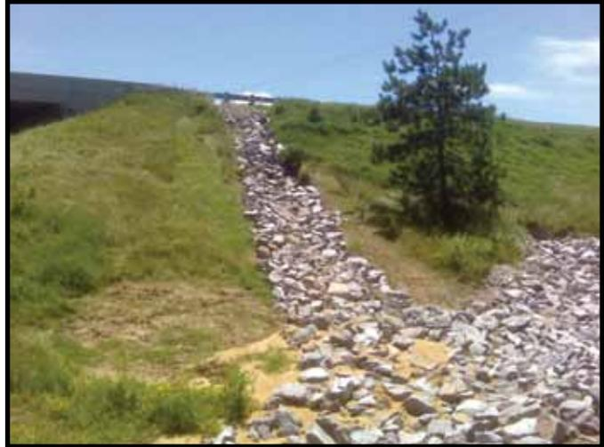
In Michigan, a highway overpass drainage outfall had repeatedly failed—to the point where the road had begun to collapse near the outfall drain outlet.
